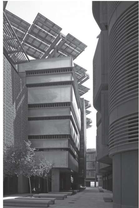
Fig. 4c: Masdar Institute: A view of a building with photovoltaic panels on the roof (2014)
