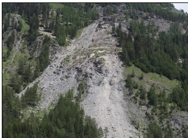
Figure 1: The Mont de la Saxe landslide (25 June 2013)
