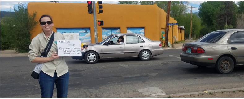
This crosswalk at Siler Road and Paseo del Pueblo Sur has a sidewalk on only one side and does not have curb ramps on either.
