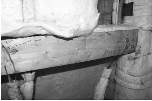
Fig. 1 Specimen placed in furnace
