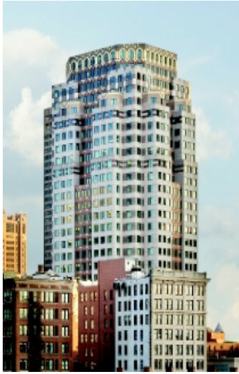
(a) Green building, MA
