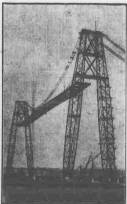
This, the second transporter in England, will be opened a few months hence. The span is 845 feet, the height of the towers 241 feet 6 inches.
