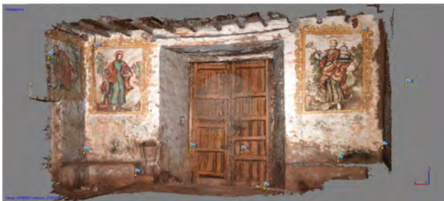
Figure 5. Final photogrammetric model of the east entrance with scaled survey points picked (blue flags) and texture applied
