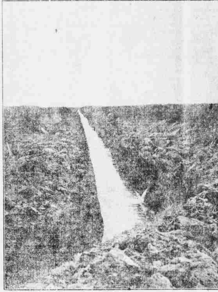
Hardwich Ditch Collecting Seepage Water for Irrigation.
