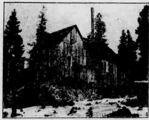
Combined Boiler and Shaft House—Tampa Mine.
