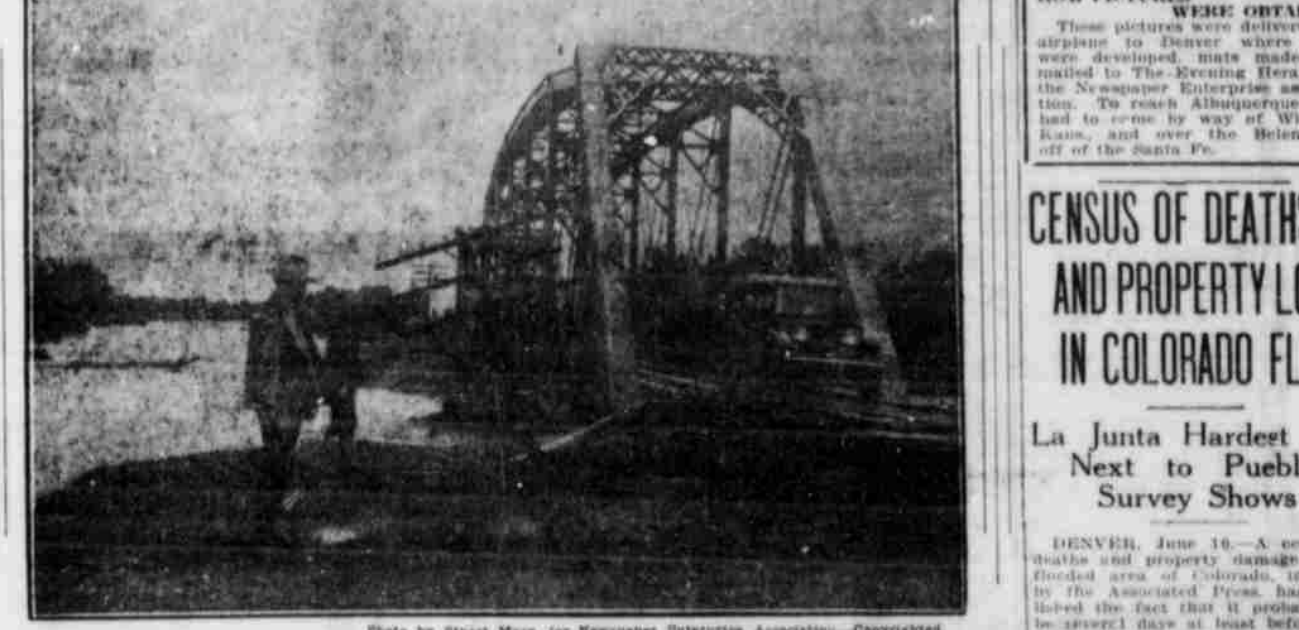
This massive Colorado and Southern railroad bridge, just outside Pueblo, Colo., was swept away by the second flood, which hit the city when Beaver Dam broke on Sunday, June 5. The concrete approaches were washed away like so much tissue paper. An auto can be seen on the railroad tracks.
