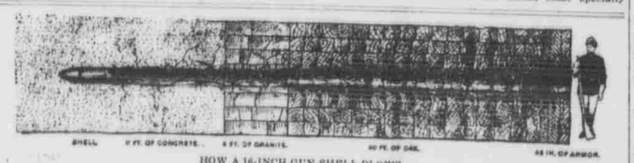
HOW A 16-INCH GUN SHELL FLOWS
