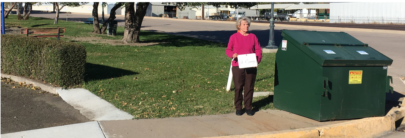
Kathryn Webb stands between a curb ramp (to her right) and a dumpster that completely blocks the sidewalk.
