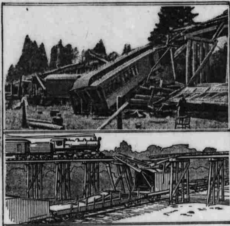
The Passenger Train Broke Through the Sagged Portion of the Trestle and Crashed on to the Work Cars Below.
