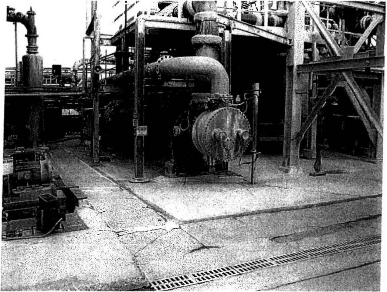
Picture No. 2, View from Southwest Corner, looking north
