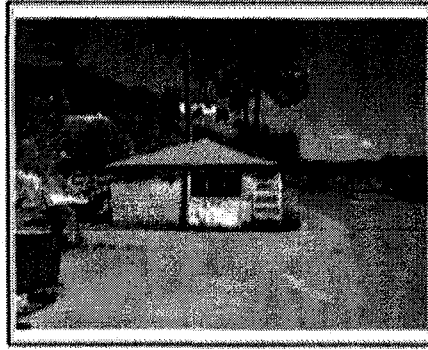
OLD STORAGE BUILDING ON PARKING LOT SITE
