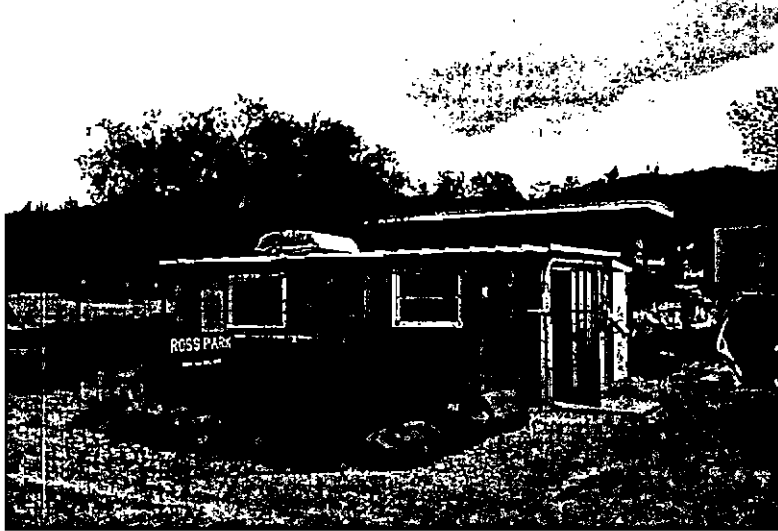
Well 28 Well House
