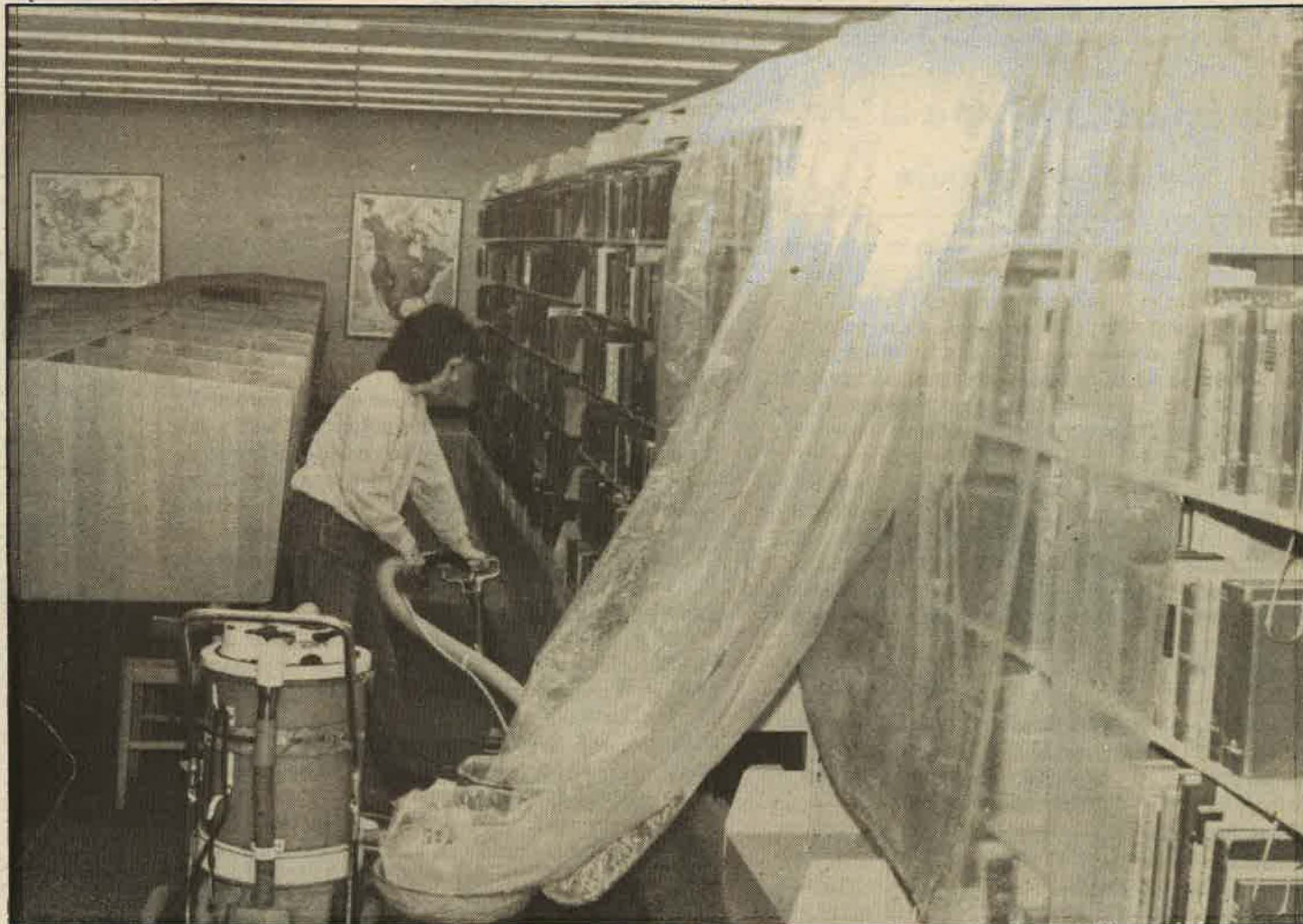
Jan Milner, custodial supervisor of Beaumont Memorial Library, Monday vacuums water on the library's second floor, after weekend rains leaked in and damaged 96 books.
