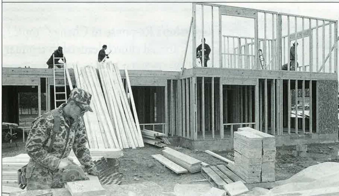
Construction has begun on the new married-student apartments located at the corner of Benton and Park streets. The complex is scheduled for completion in August by the beginning of the fall semester.
