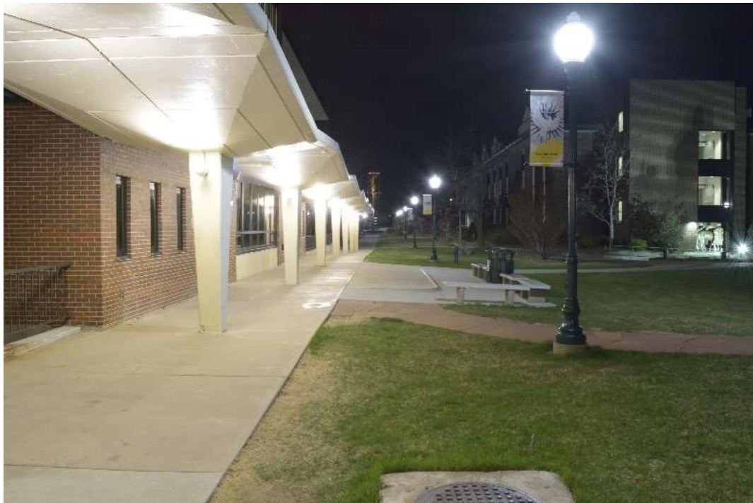
Figure 21: Redundant accent lighting outside DeSmet Hall
