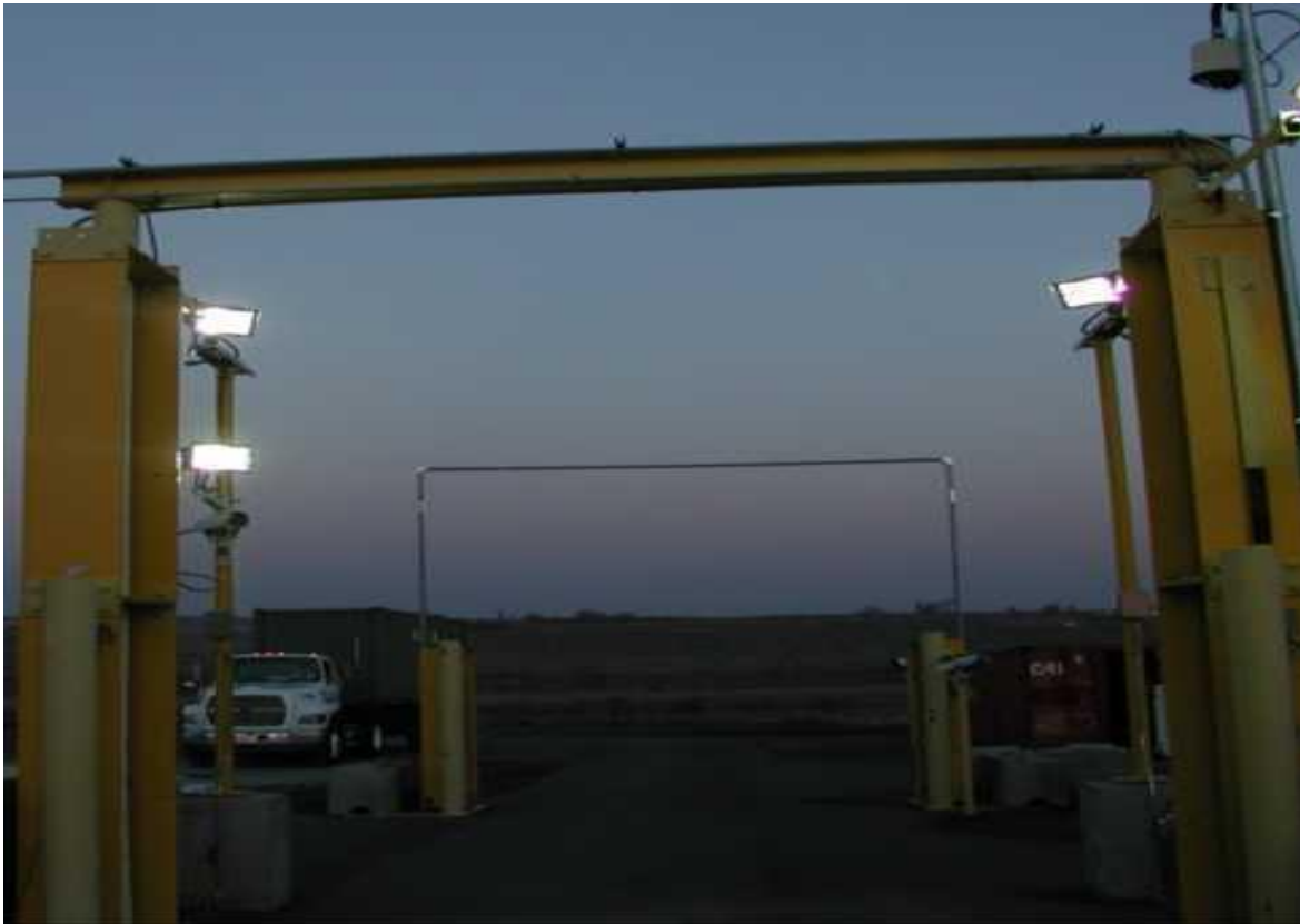
Figure 12: Light Fixture Placement for Rear Image Testing
