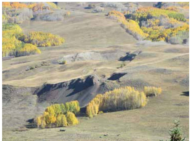
Barren shale is exposed where rock has slumped away from the hillside. The uneven slopes on the hillside above result from soil movement. Photo by Tom Zeiner.
