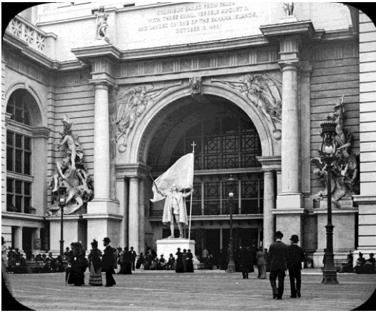
Figure 6: Detail of Administration Building Entrance
