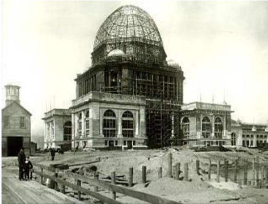
Figure 2: Construction of the Administration Building, 1893 Columbian Exposition
