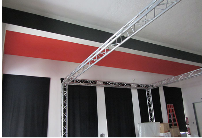
Figure 3.50. Hinnerk Scheper, Detail, Canteen in Festive Wing, in Walter Gropius' Bauhaus Building, Dessau, 1926 (Color Restoration, 1996-2006) (Photo: M. Ridler, 2013).
