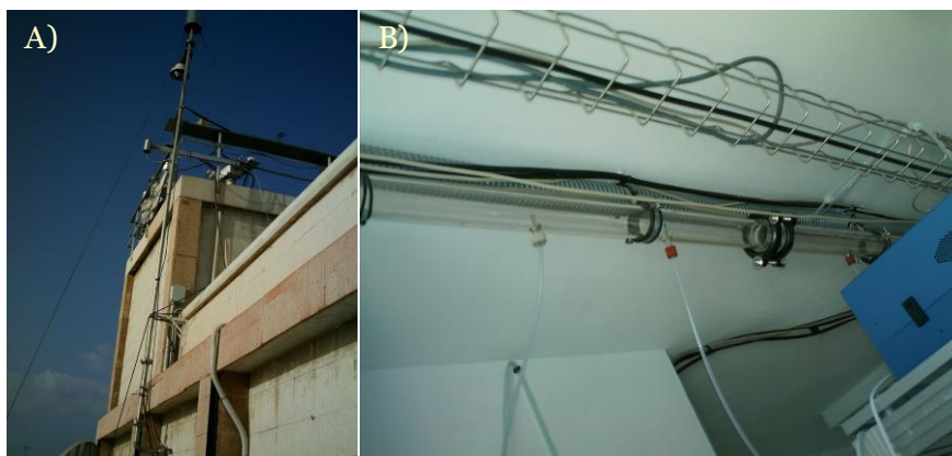
Figure 2.8 A) Design of the sampling inlet line and B) manifold at SCO
