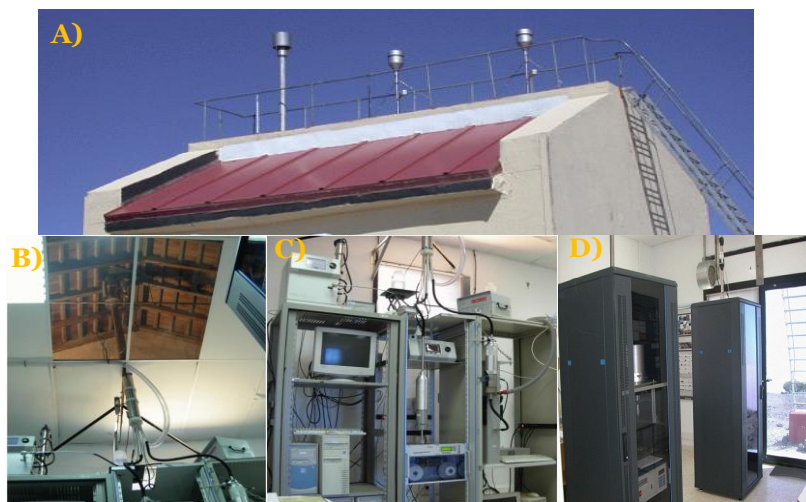
Figure 2.24 Inlets (A) and indoor view (B-D) of the PARTILAB at IZO
