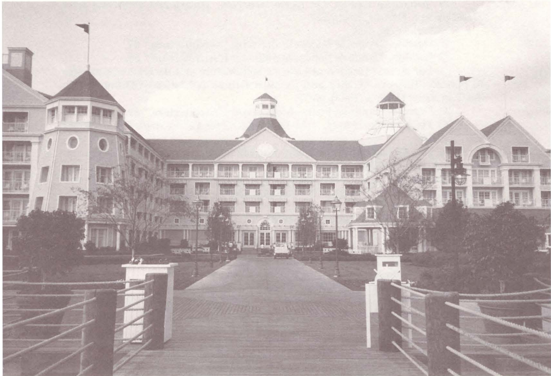
Figure 1: Disney resort designed by Robert A. M. Stern, a recent example of Pomo architecture. It is a recreation of past "homey" images constructed by applying advanced building technology: plastic columns, imitation wood siding, etc., as a representation of Disneyesque high-profile commodity.
