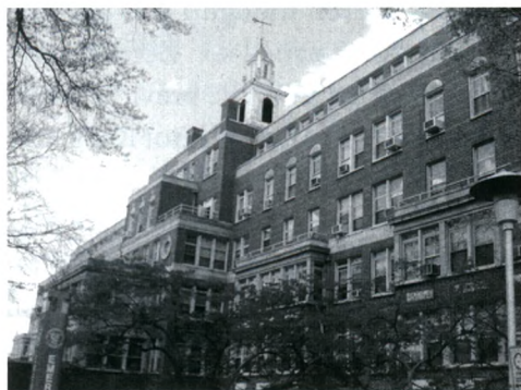
Figure 14C: The Munger Pavilion at NYMC, is a former tuberculosis sanatorium, housed my administrative office for 15 years.
