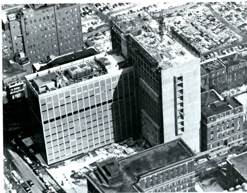
Figure 8B: The construction of the Boston University School of Medicine instructional building, finished during my senior year (1968-1969). At right are the old buildings where I took my basic science courses. The Pavilion Building at Boston City Hospital, where I completed my third and fourth year medicine rotations is in the foreground. In the rear is University Hospital where I completed my fourth year surgery rotation. (Image courtesy of Boston University. Reprinted with permission.)
