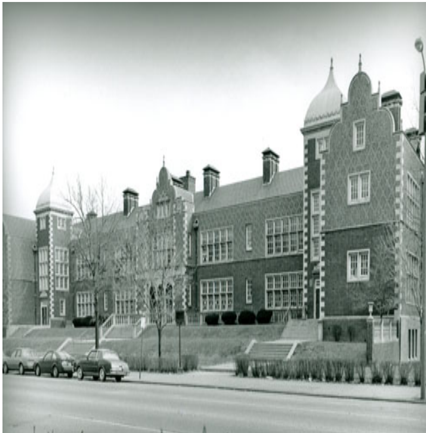
Clark Elementary School (now closed) 1020 Union Boulevard, built 1906
