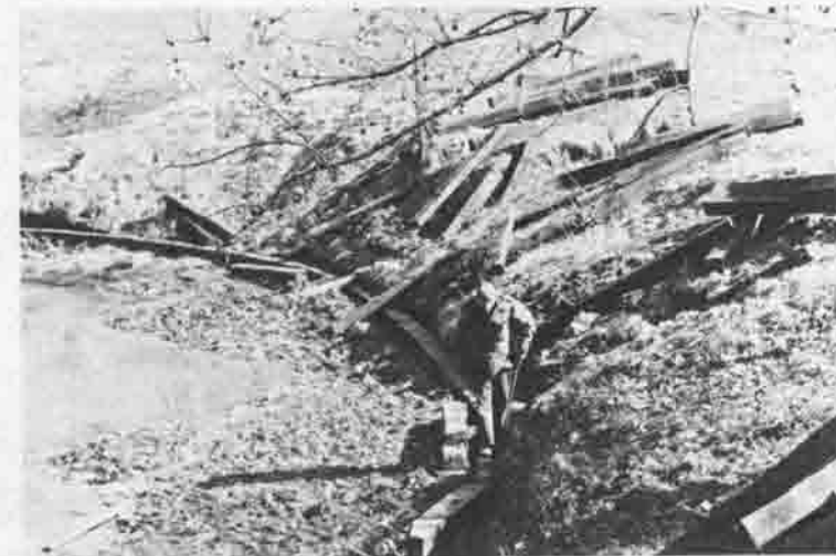
Workers are shoring up the banks of Bugg Lake with railroad ties in an effort to stop erosion.
