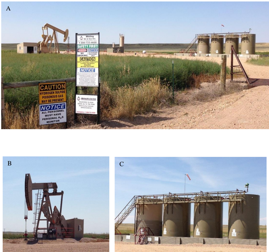
Figure 2. Example oil and natural gas site infrastructure on the Pawnee National Grassland. A = Full site, B = pumpjack, C = condensate tanks, D = Evaporation pit, E = older tank and stack.
