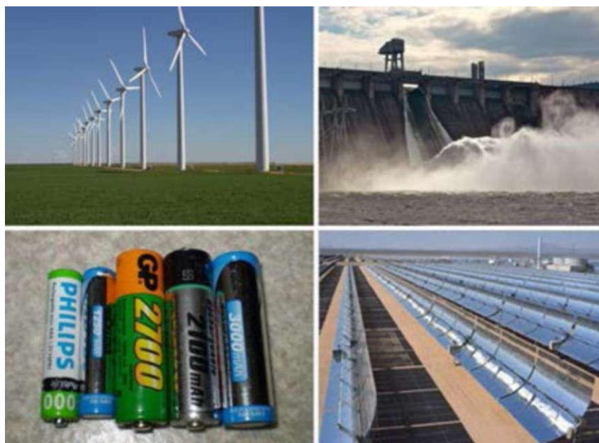
Figure 5.1 A variety of voltage sources (clockwise from top left): the Brazos Wind Farm in Fluvanna, Texas (credit: Leaflet, Wikimedia Commons); the Krasnoyarsk Dam in Russia (credit: Alex Polezhaev); a solar farm (credit: U. S. Department of Energy); and a group of nickel metal hydride batteries (credit: Tiaa Monto). The voltage output of each depends on its construction and load, and equals emf only if there is no load.
