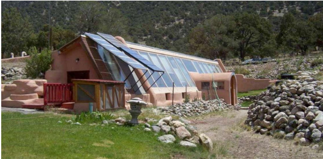
Figure 5.5. Passive solar building near Crestone, Colorado (image from Wiki Commons)
