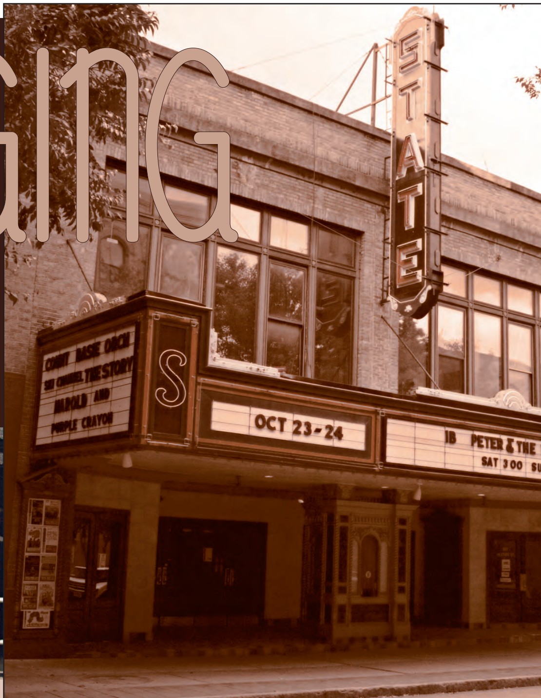
The State Theatre, located at 107 W. State St., has been a part of the Ithaca community since its opening night in 1928. Thirteen years ago the theater was in danger of being torn down because of structural damage. KELSEY O'CONNOR/THE ITHACAN
