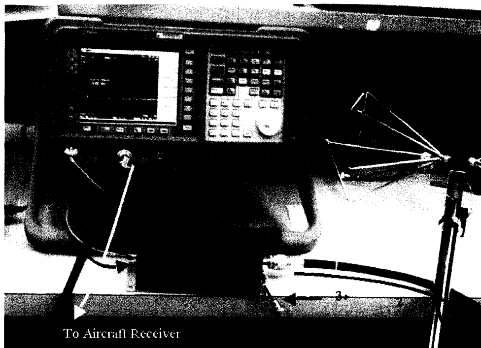
Figure A.6. Complete hook-up of Spectrum Analyzer with power-amp, coaxial cables, transmitting antenna and laptop computer.
