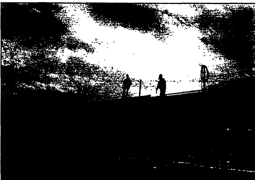
CONSTRUCTION WORKERS on the roof of the half-completed fitness center. The center is the only building project at Ithaca College currently on schedule.
