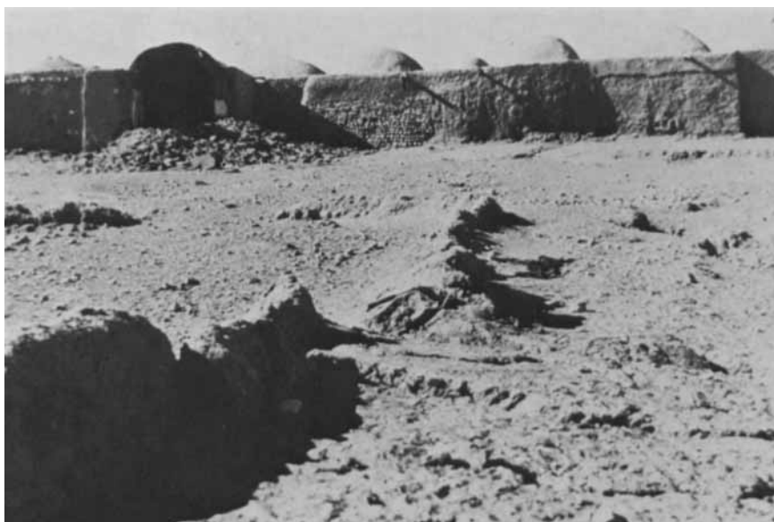
Figure 11. A 0.9 m right-lateral displacement following the Kurizan earthquake. The displacement is measured from boundaries of land parcels. Note that the adobe building about 100 m from the fault trace which is nearly parallel to the wall did not collapse. This indicates that ground acceleration produced by this event is not very high.
