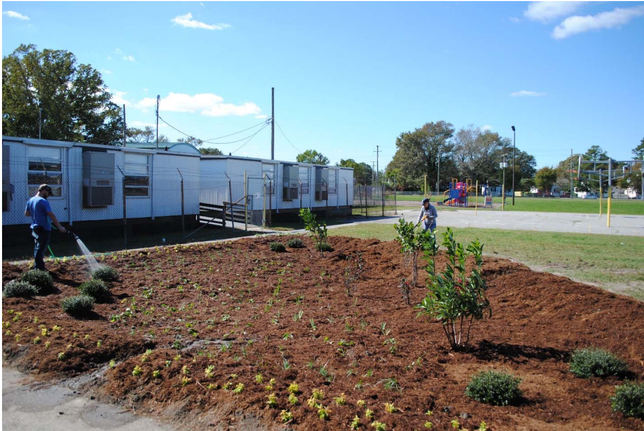
Figure 1. Rain garden implementation project.
