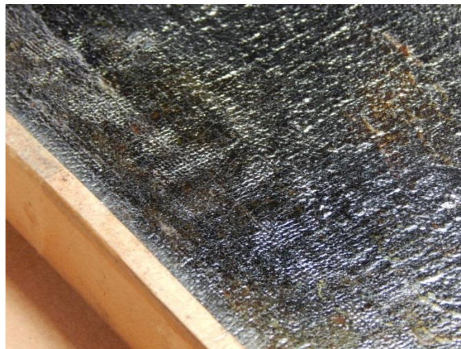
Figure 5. Detail of imprinted weave pattern along the length of a crack. The pattern appears to have been intentionally added to disrupt the smoothness where the cracks were blended.
