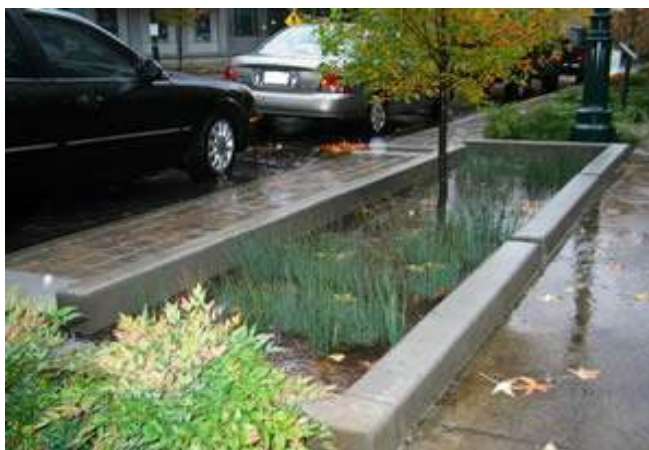
Figure 9-A.2. Expanded Tree Pits
