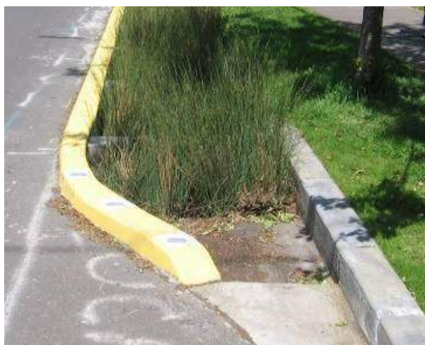
Figure 9-A.3. Stormwater Curb Extensions
