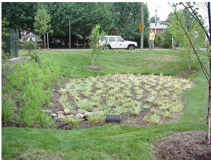
Figure 9.1. A typical Bioretention Filter treating a commercial rooftop
