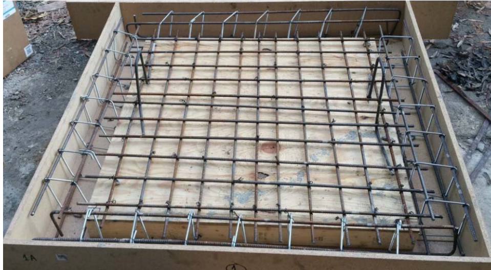
Figure 43. Reinforcement skeleton in formwork for slab specimens
