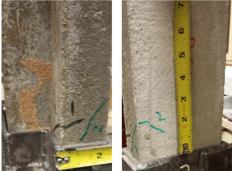
Figure 83. Final crack pattern of SM11
