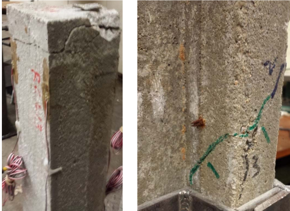
Figure 89. Final crack pattern of SM13
