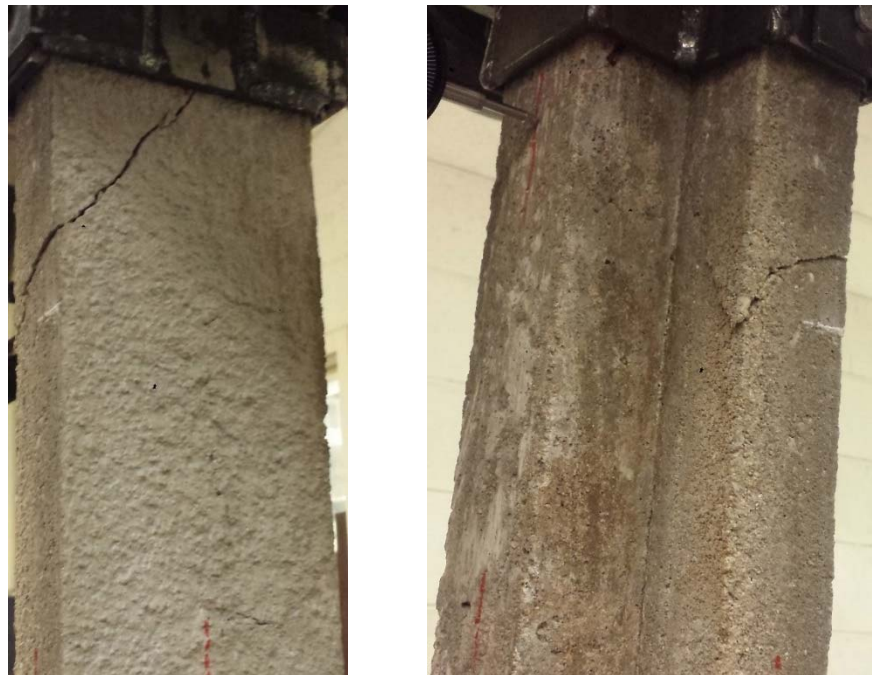
Figure 74. Final crack pattern of SM07
