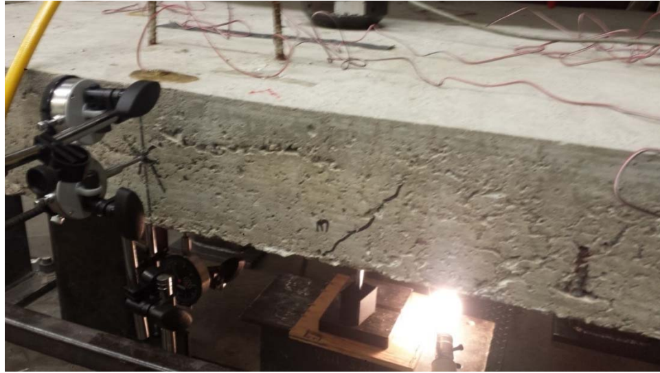
Figure 108. Cracks in spandrel member of SL01 at a load of 25.72 kip
