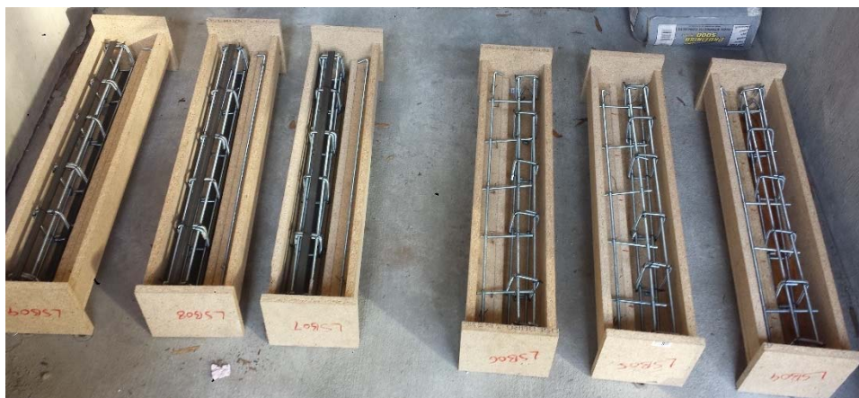
Figure 42. Formwork with reinforcement for spandrel members
