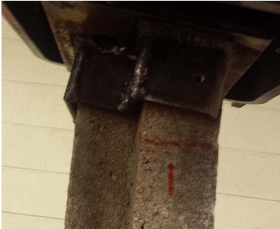
Figure 71. Final crack pattern of SM06
