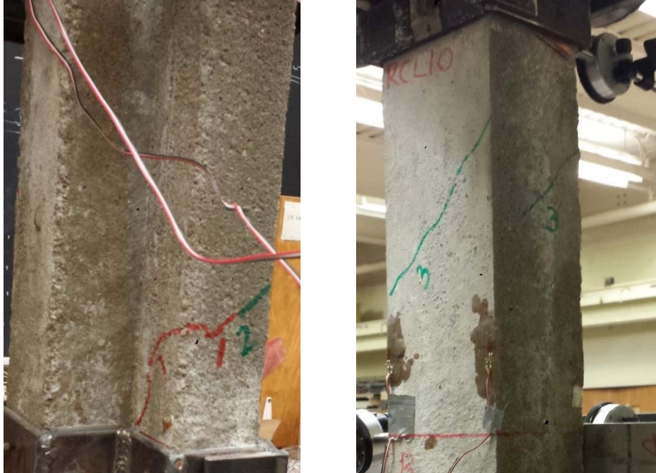
Figure 76. Final crack pattern of SM08
