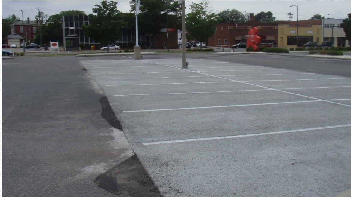
Figure 1. Pervious concrete parking area sampled at the Science Museum of Virginia from November 4-December 30, 2013.
