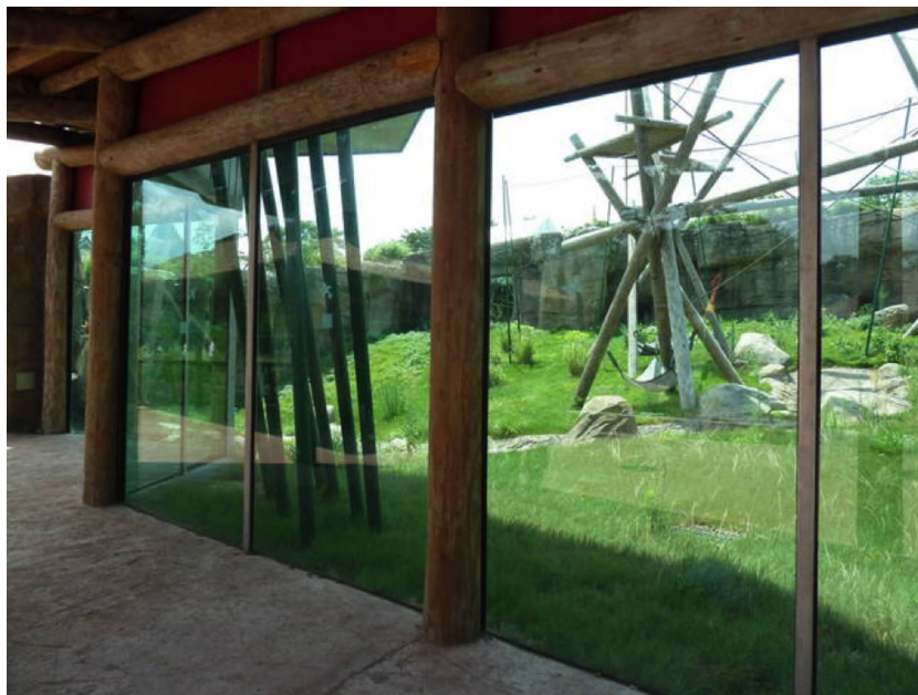
Figure 1 Typical view of exhibits associated with high window-strike fatalities, showing habitat beyond large, transparent glass panes.
