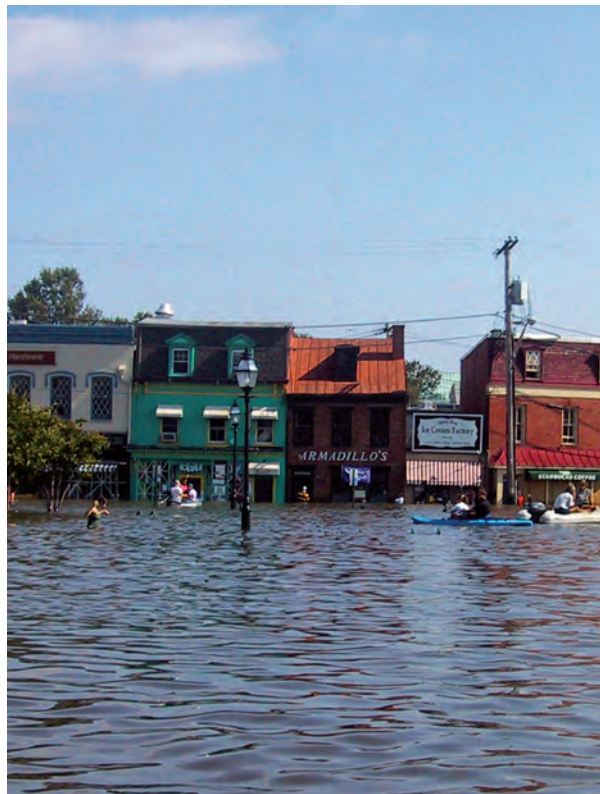
Downtown Annapolis was flooded during Hurricane Isabel in 2003. Higher sea levels will increase the extent and frequency of flooding from such storms.
