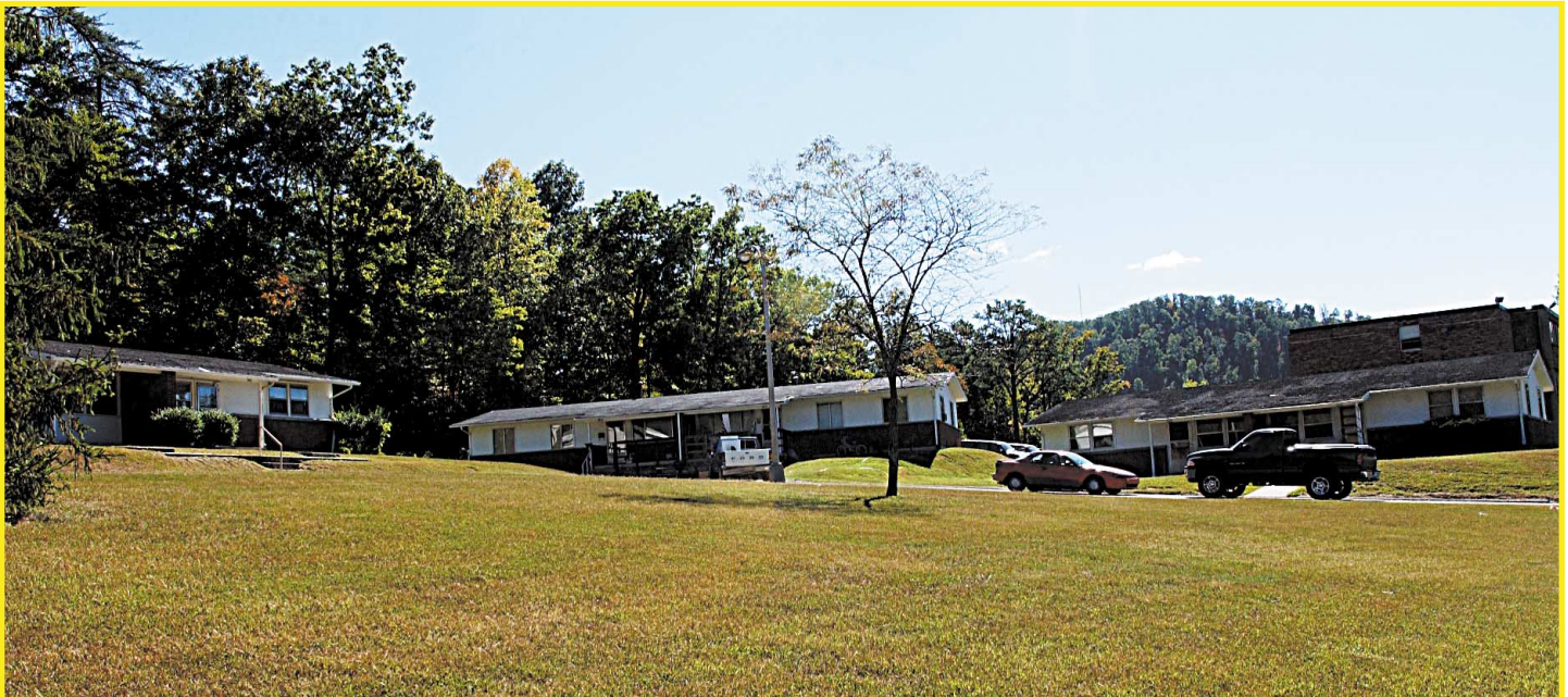
These 40 year-old apartment buildings in Lakewood Terrace will be renovated to become the temporary support facility for the Space Science Center antenna system.
