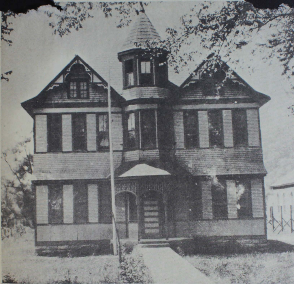
Salyersville Grade School, replaced by brick school in 1936
