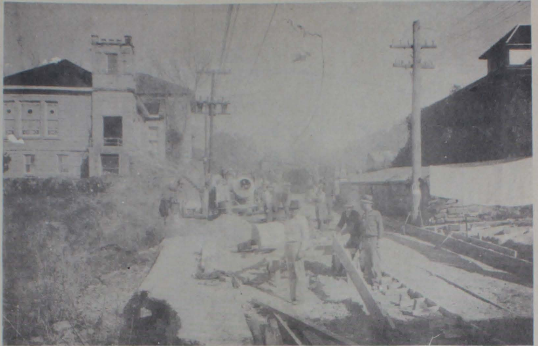
THE BUILDING OF CHURCH STREET. . . Goldie Prater provided this photo taken while WPA workers were building Upper Church Street in Salyersville. To the left is the Christian Church.
