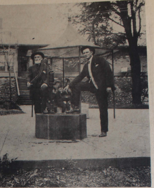
Arcadia Well With Railroad Depot (Present Legion Park) In Background
