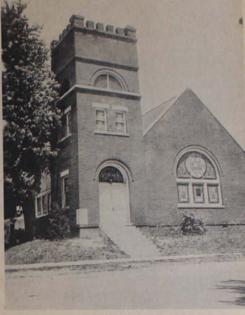
First United Methodist Church Building Used Until 1970
