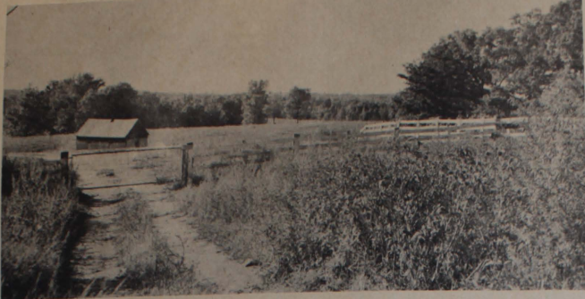
Once A Field, Now Clarkdale Court
