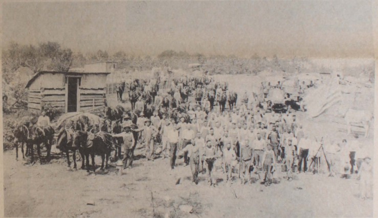
Outwood Construction Begins
