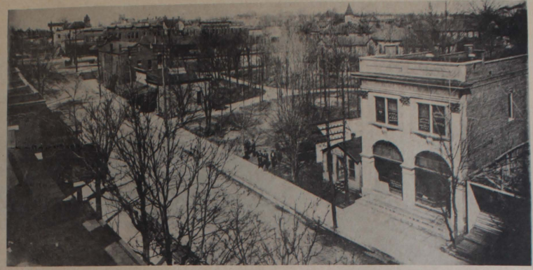
In Early 1900s Downtown Dawson Springs Already Had Nice Business Buildings
