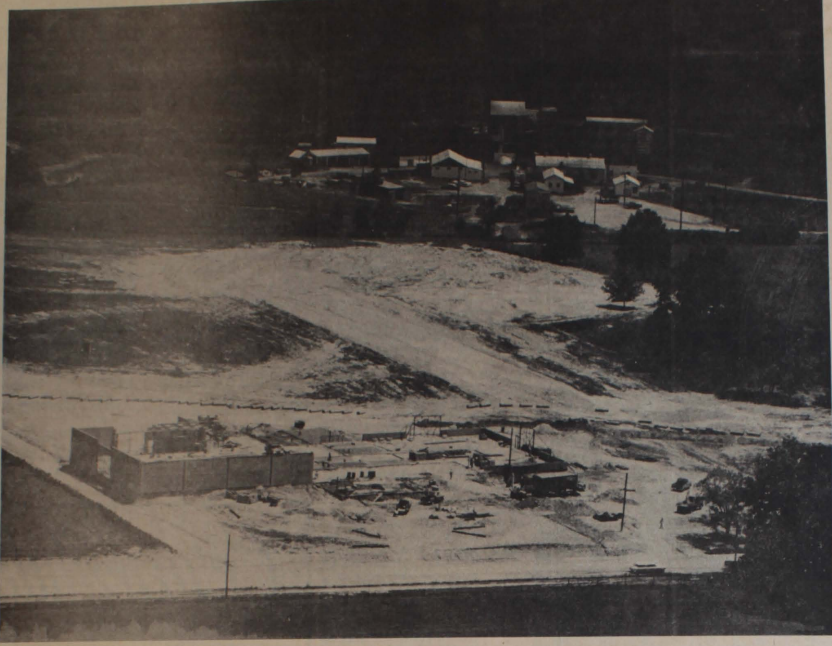
Mid-South Plastics Building Starts In 1963; Dawson Collieries In Background
