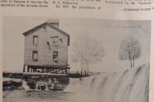
Old Mill Dam On Tradewater River
