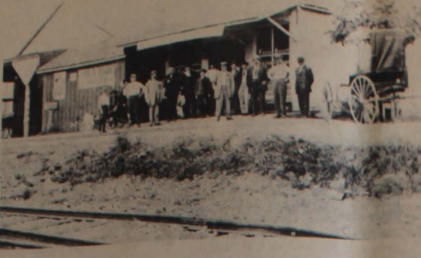
IN 1909, HORSE AND BUGGY carried passengers to Mount Washington and ended shortly beyond this point in Fern Creek.
