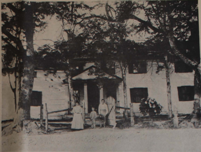
former Margaret Fegenbush, who was married to Edward Vogt. Miss Vogt stressed the fact that, although the land they own is the original, the houses are not.
