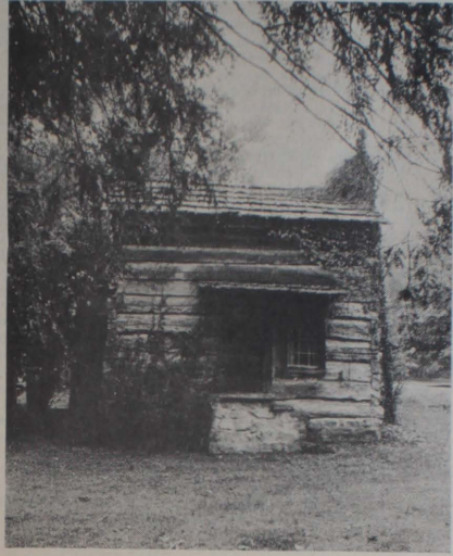
Uncle Solomon Everidge's cabin was moved to the campus in 1930.
