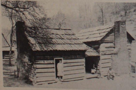
Dogtrot log cabin pictured around 1900 was similar to housing in the county during the Civil War.
