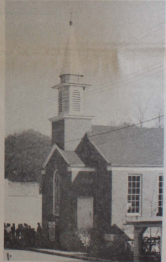
Church which burned in 1979. Built 1948.
