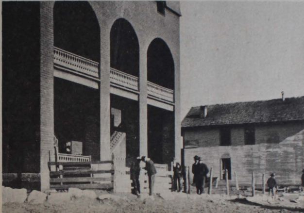
The Knott County Courthouse (in the 1890s) before the work on its exterior and the grounds was completed. Note that the fence posts are up but that the fence is not completed.
