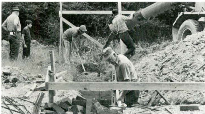
W. H. Rice supervises the excavation as work begins.
