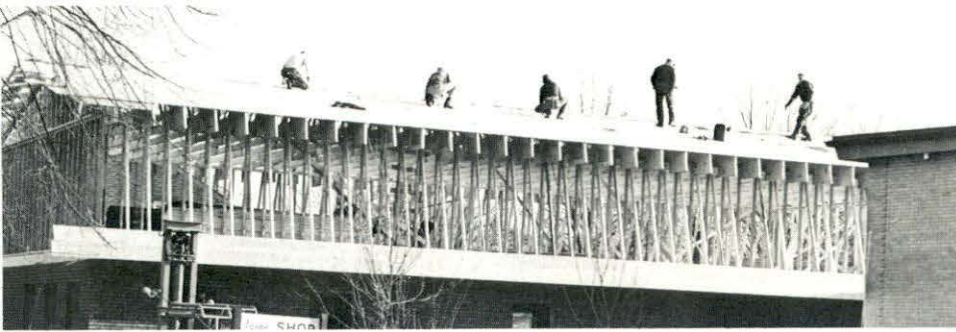
The second floor takes shape as workmen continue rapid progress.
