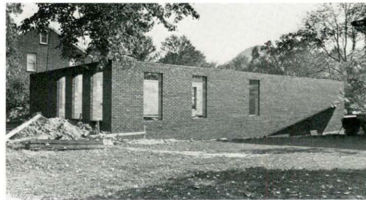
Brick and block reach the second floor level.
