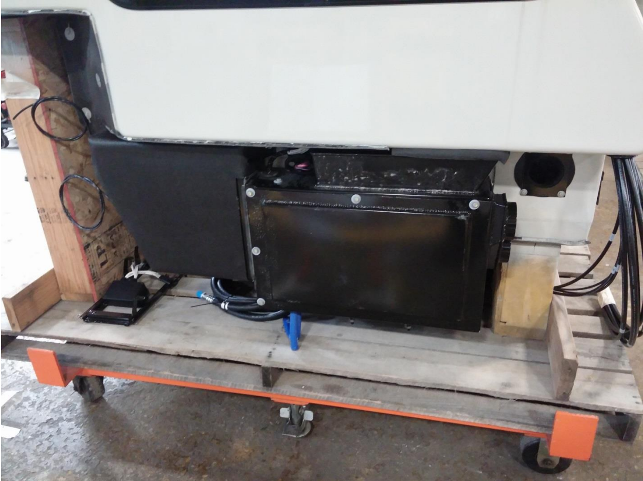
Photo of actual HVAC enclosure installation
