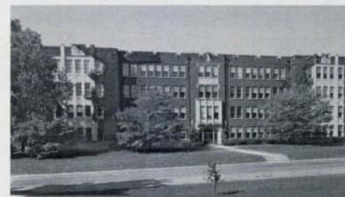
Figure 4. Lappin Hall before two additions.
