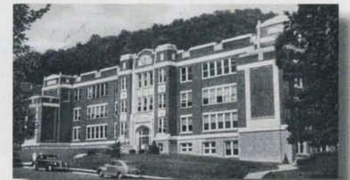
Figure 10. Original Breckinridge Training School before two additions.
