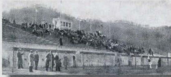
Figure 12. Old concrete Football Stadium.
