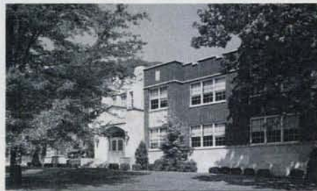
Figure 11. Original Baird Music Hall before two additions.
