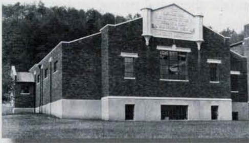
Figure 5. Senff Natatorium before demolition.
