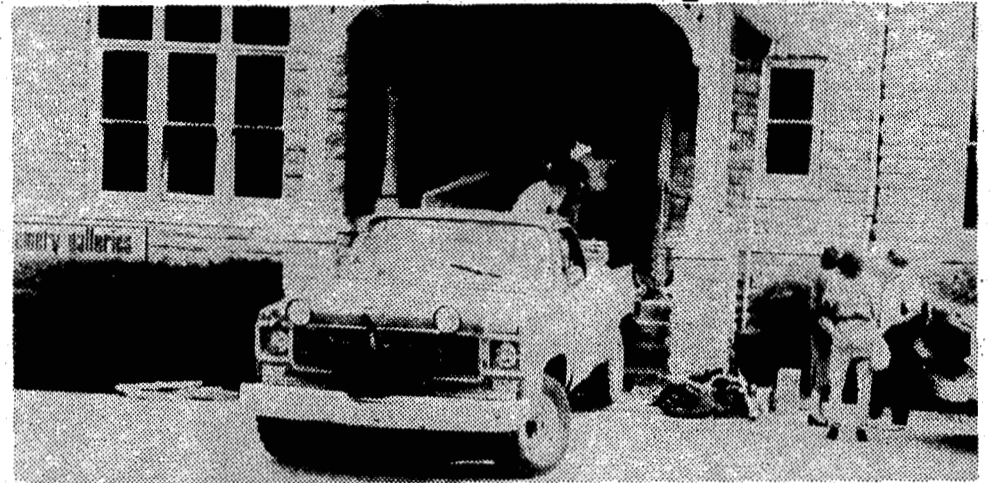
Construction workers removed pieces of Italian marble tile from Emery during the protest on Sept. 20.
